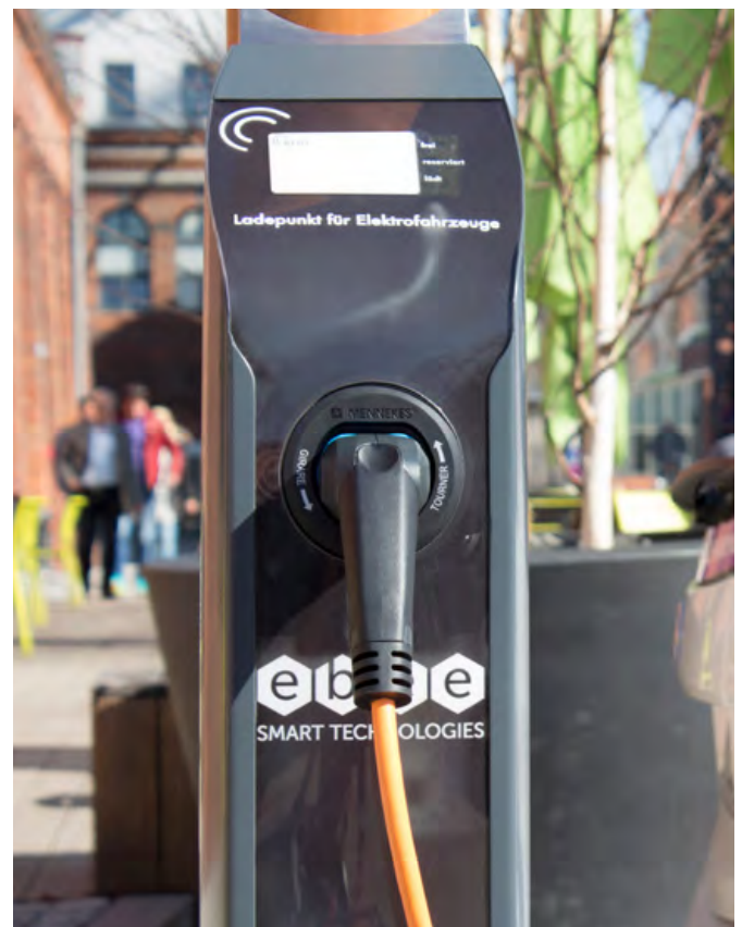
Ebee charging point: user identification and authentication via RFID or app.
