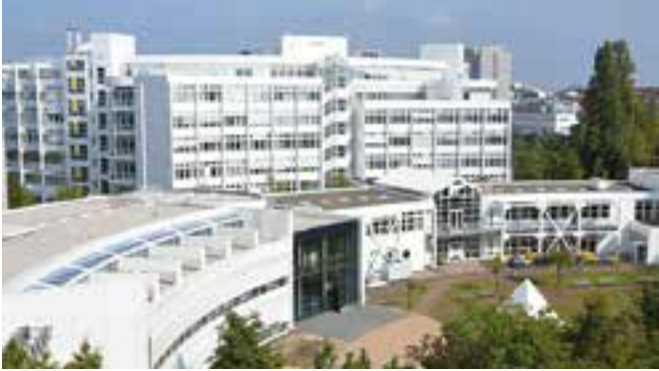
Production Technology Center (PTZ) Berlin, left in the foreground the new Microproduction Technology Application Center (AMP) © Fraunhofer IPK
