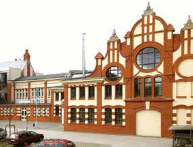
PTB in Berlin Charlottenburg: the Imperial Metrology Institute was founded here in 1887 under Hermann von Helmholtz. © Physikalisch-Technische Bundesanstalt
