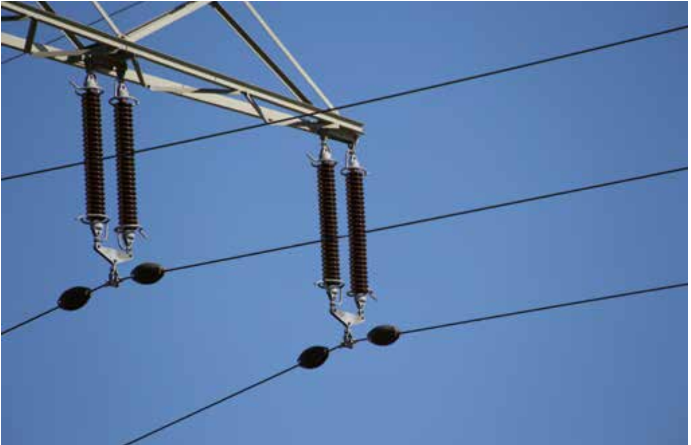
The wireless sensors below the insulators enable the monitoring of high and extra-high voltage lines.
