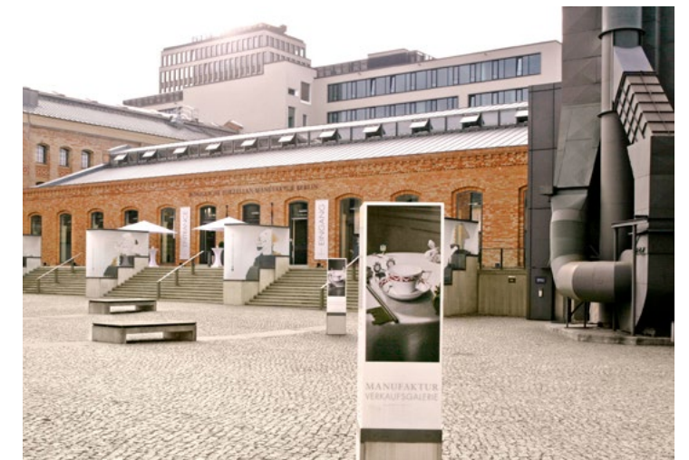
Today, the historic kiln hall functions as a sales gallery.
