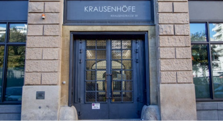
The Krausenhöfe (Krausen Courtyards) are home to Amazon's Berlin development center
