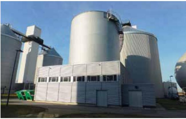
Berliner Wasserbetriebe plant where magnesium ammonium phosphate (MAP) is recovered from sewage sludge
